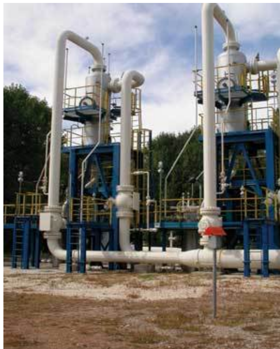
In order to protect its downstream system from black powder, DEPA installed two cyclone (centrifugal) filtration facilities at the start of its network next to the Bulgarian border. Use of these filters enhanced the effectiveness of trap filters further downstream (Fig. 6).
