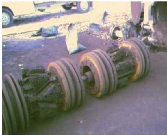
Dual module bidirectional pigs with brushes continued to remove large amounts of black powder even after other techniques had been applied. The interior of the pipeline on the Bulgarian side of the border was not protected with coating (Fig. 4).
