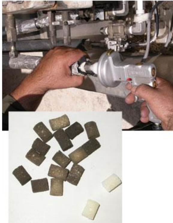
A pellet launcher (left) removed black powder from gas metering impulse lines. The pellets used (right) turned black after just one pass through the impulse line (Fig. 7).
